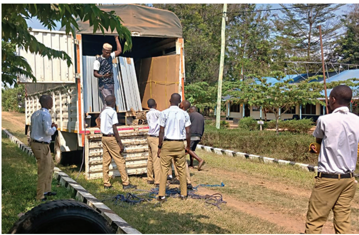
Work team unloads solar panels to install them at Tumaini.
