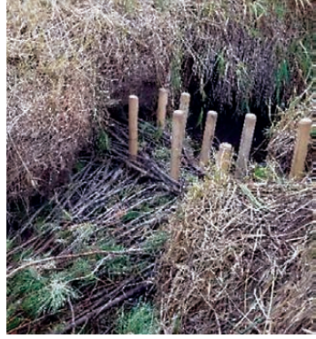
Thompson Creek BDA Restoration Project paper shows posts driven into the creek and pine branches that will be woven around them.
