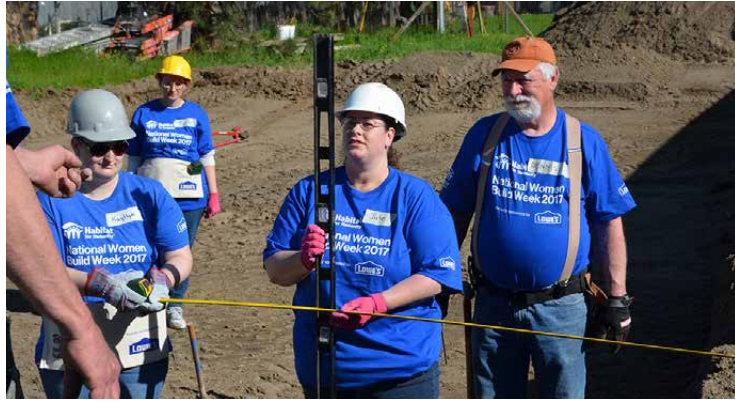
North Idaho Women's Build volunteers prepare for foundation.
