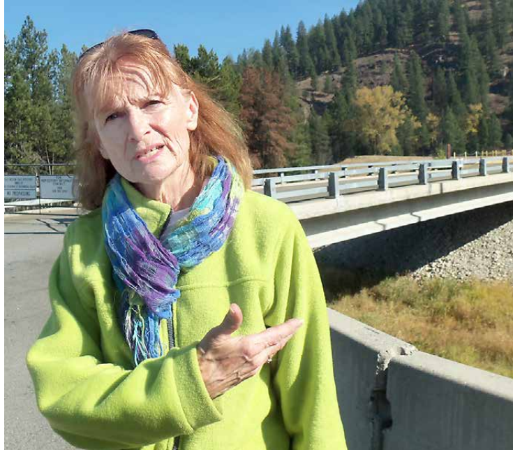
Barbara Miller visits contaminated site near Cataldo Mission.
