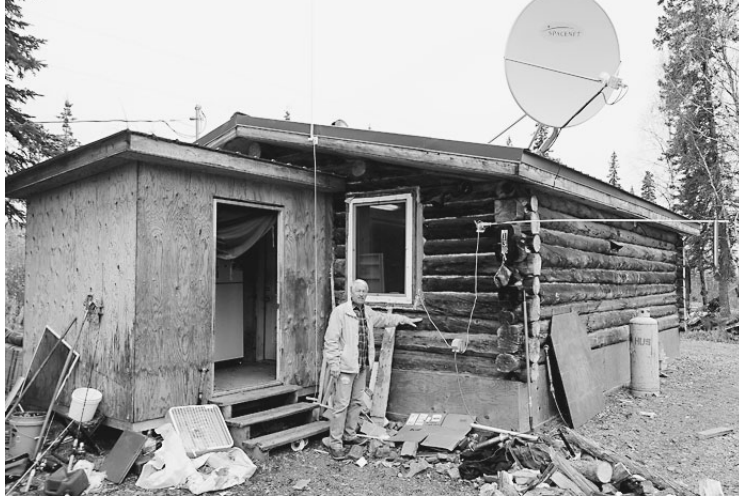
David Helseth's hand is at the level of floodwaters.
